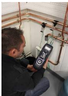
DHW network temperature
