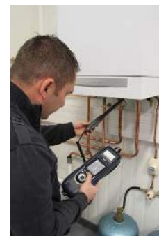
Ambient CO checking
